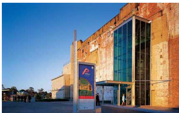
Brisbane Powerhouse, New Farm Park
